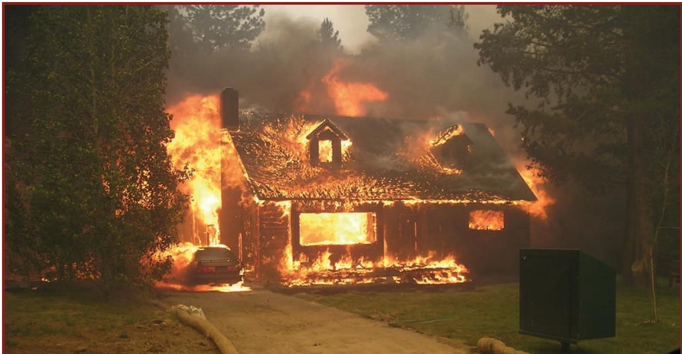
**Figure 9.** Note the unburned vegetation immediately adjacent to the structure indicating the ignition was from a spot fire.
