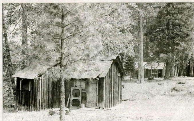
Richard Jacks originally settled the Meadow Valley property the Forbes now own. Crews cleared brush and vegetative debris from around the old cabins, not only to help save them, but to help reduce the fire danger. The dry timber would easily ignite if a spark landed in nearby brush or pine needles.
